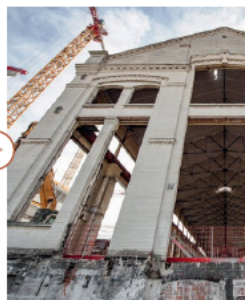
2020: START OF WORKS Development and redevelopment of the wasteland
